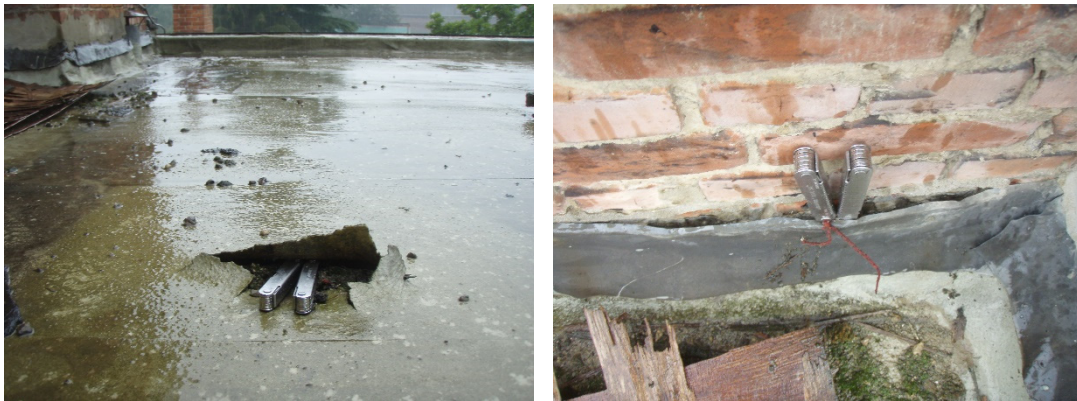
Fig. 2 – Infiltrations in roof surface and connections, 2011.
