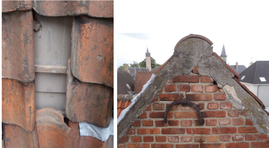
Fig. 4 – Left: uncovering of roof sheathing and pan laths due to shifting of tiles, 2015. Right: deterioration at connection raised gable due to incompatible cement based mortar, 2015. Pictures by MOWAv.
