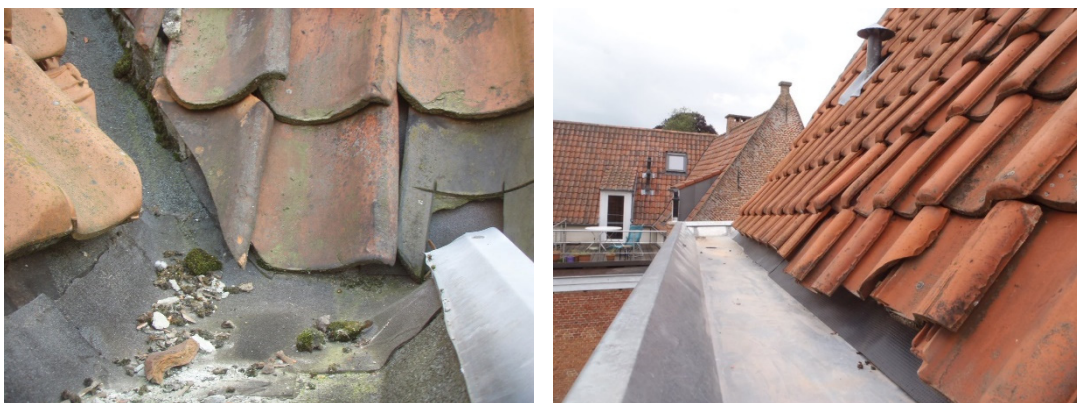
Fig. 3 – Left: gutters in asphalt, 2011. Right: new gutters with zinc linings, 2015. Pictures by MOWAv.
