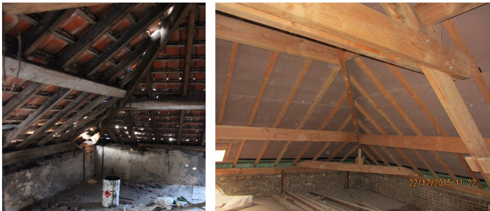
Fig. 1 – Left: roof structure before renewal, 2013 (picture by owner). Right: roof structure after renewal, 2015.
