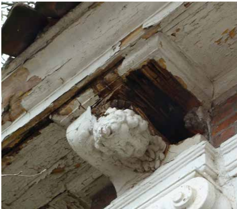
Figure 3.2.1 Moisture led to wood rot and loss of material of the console
