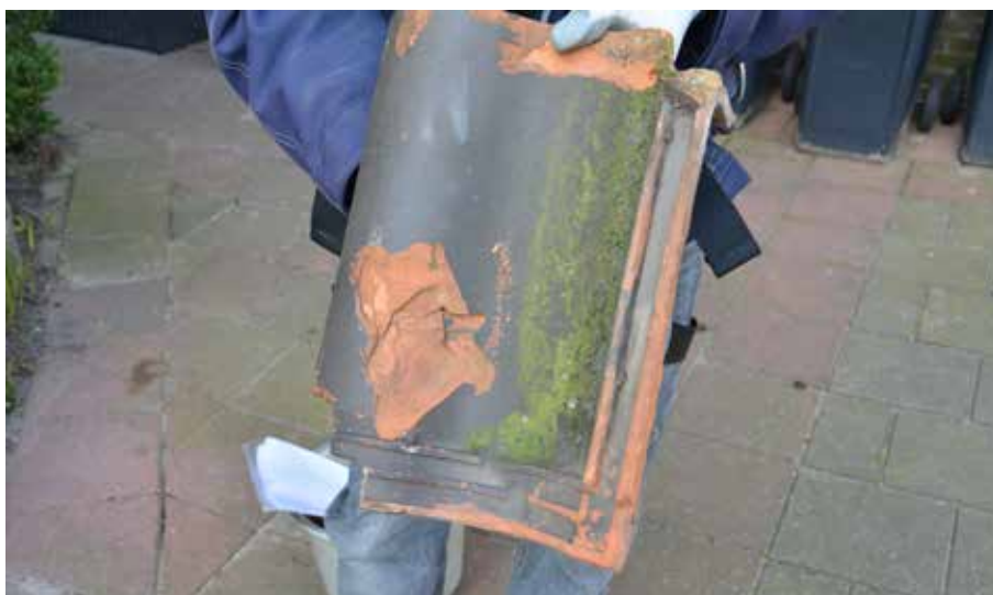
Figure 5.1 Pushed out pointing. Annoying, but it is a problem that can be tackled in the medium-long term
