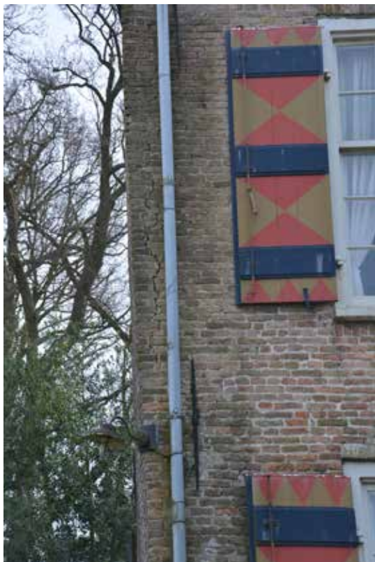
Figure 4.3.2 Long crack at the connection of a side and an end facade (drawing from a student report, June 2015) [5]
