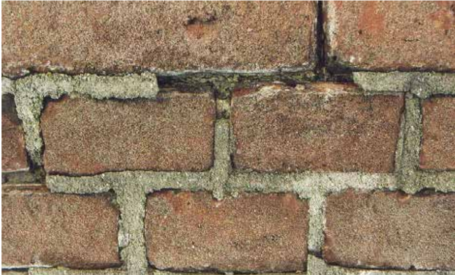
Figure 3.3.3 Pointing being pushed out
