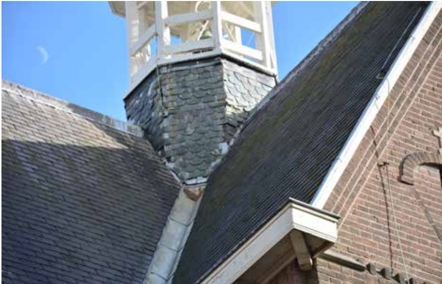
Figure 4.1.1 a/b Overdue maintenance of the chapel identified by the inspection of MW: paintwork in bad condition, wood rot, missing slate tiles
