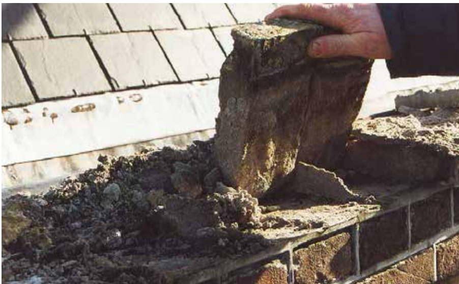
Figure 3.3.4 Crumbling and complete disintegration of the bedding mortar
