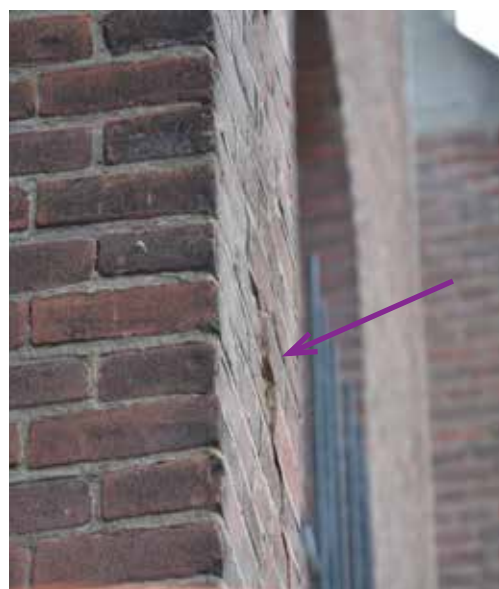
Figure 4.1.2b The photo shows a buttress with a piece of masonry that came loose, making visible a rusting anchor. Figure 4.1.2c The photo shows that here as well a piece of masonry is getting loose and being pushed out. Both cases show a potentially dangerous situation
