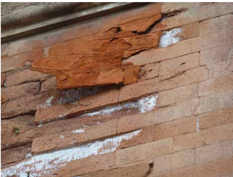
Figure 3.1.2 Loose parts of masonry, posing potential danger for passers-by
