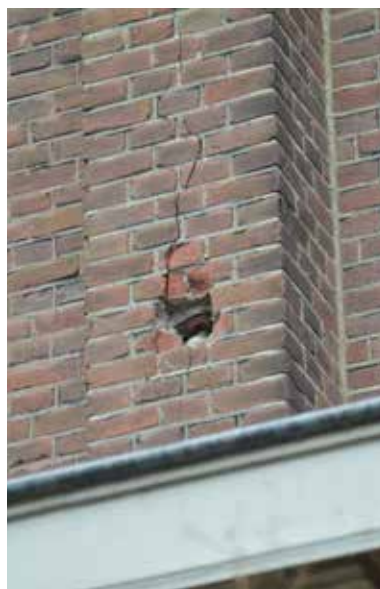
Figure 4.1.2b The photo shows a buttress with a piece of masonry that came loose, making visible a rusting anchor. Figure 4.1.2c The photo shows that here as well a piece of masonry is getting loose and being pushed out. Both cases show a potentially dangerous situation
