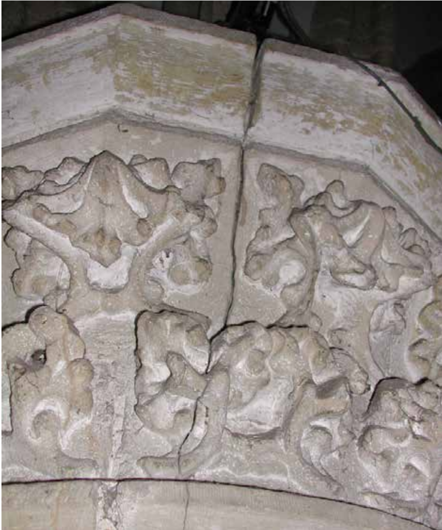
Figure 3.1.1 Cracked capital, which might lead to a dangerous situation
