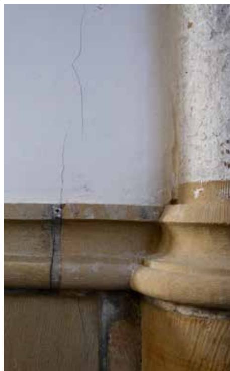
Figure 3.4.1 Crack formation in masonry and monitoring of masonry. It is important to determine whether it is a foundation related or other structural problem and also whether settlement still occurs
