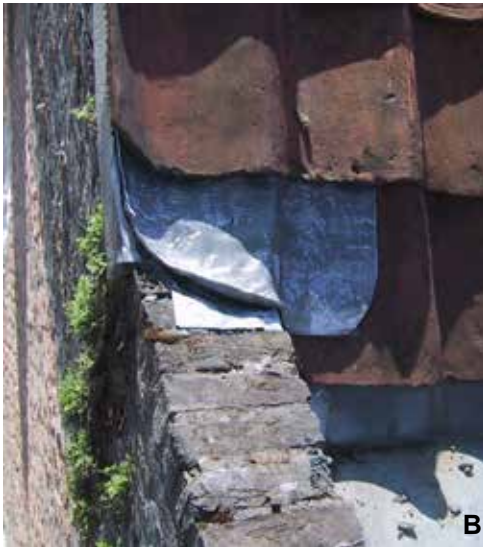
tween roof and façade (a. As encountered; b. Improved; c. Condition two years later)
