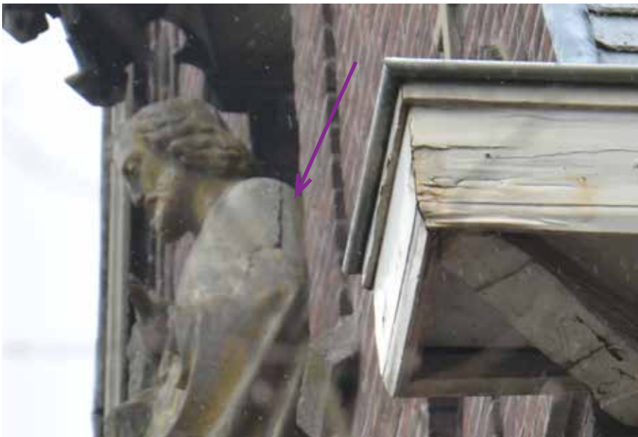
Figure 4.1.2 a The sculpture clearly shows a crack
