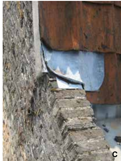
tween roof and façade (a. As encountered; b. Improved; c. Condition two years later)
