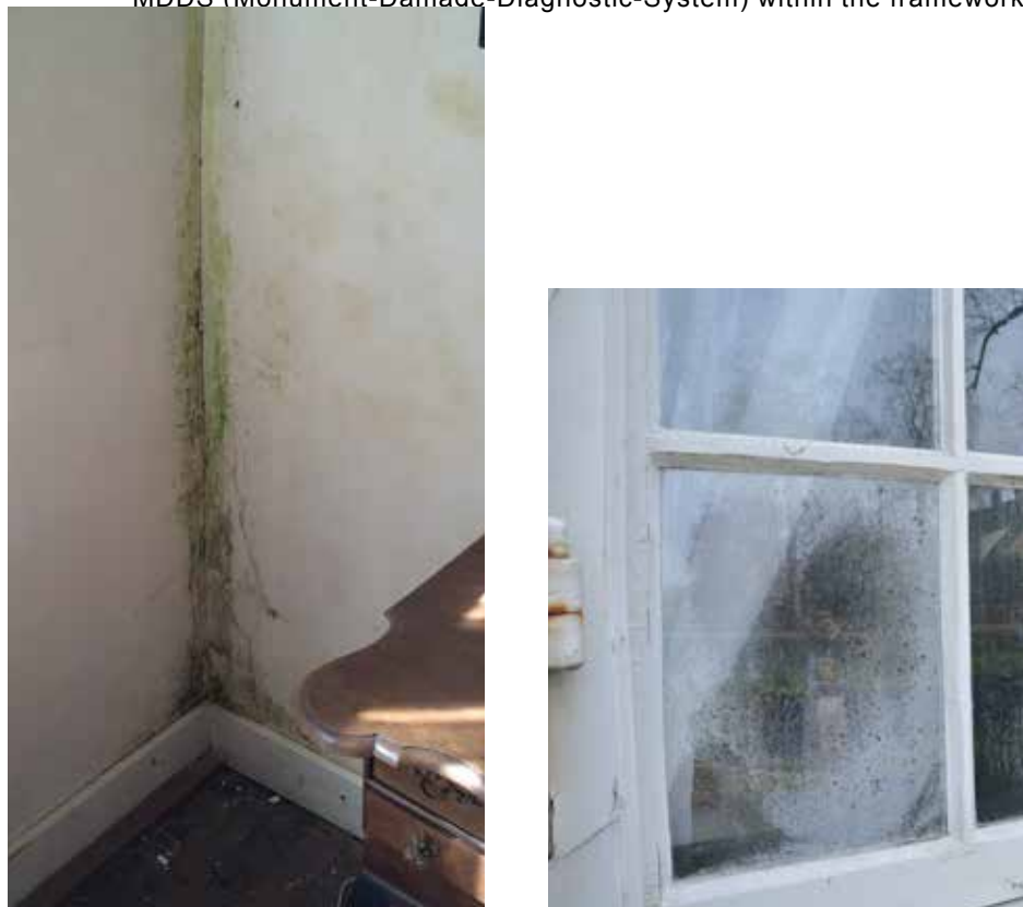
Figure 4.3.3 Moisture-related problem on the inside of the façade, reflected by algae growth. The problem lies at the location of the previously mentioned situation (continuous crack and problem with rainwater drainage) shown in Figure 4.3.2 (l). The sometimes high air humidity leads to condensation on the glazing (r)
