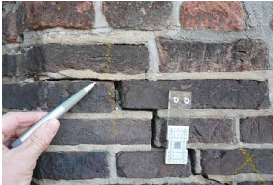
Figure 3.4.1 Crack formation in masonry and monitoring of masonry. It is important to determine whether it is a foundation related or other structural problem and also whether settlement still occurs
