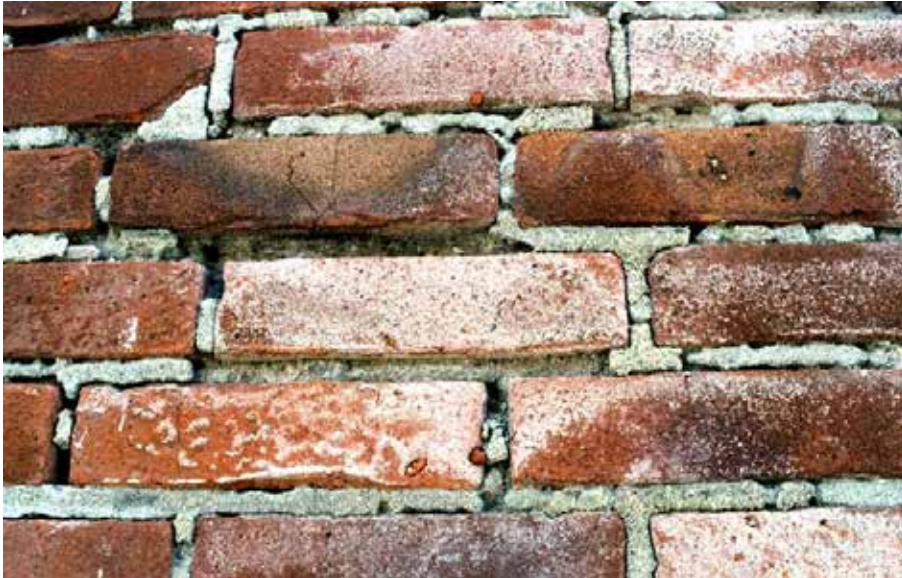
Figure 3.2.3 Moisture and salt problem, resulting in damage to pointing mortar and bricks
