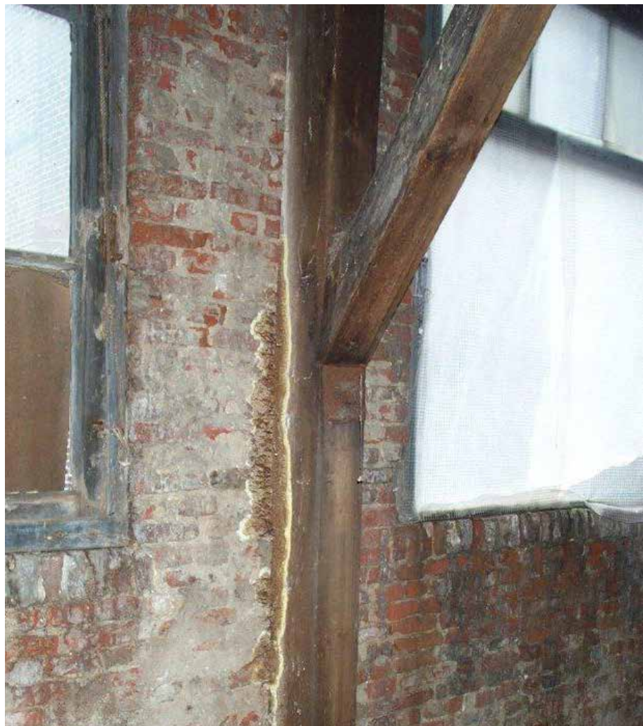
Figure 3.2.2 Infestation of the wooden wall baluster through dry rot fungus, as a result of long-term exposure of the wood to water penetration. The consequence is that in this case the entire wood construction had to be removed ('worst case')
