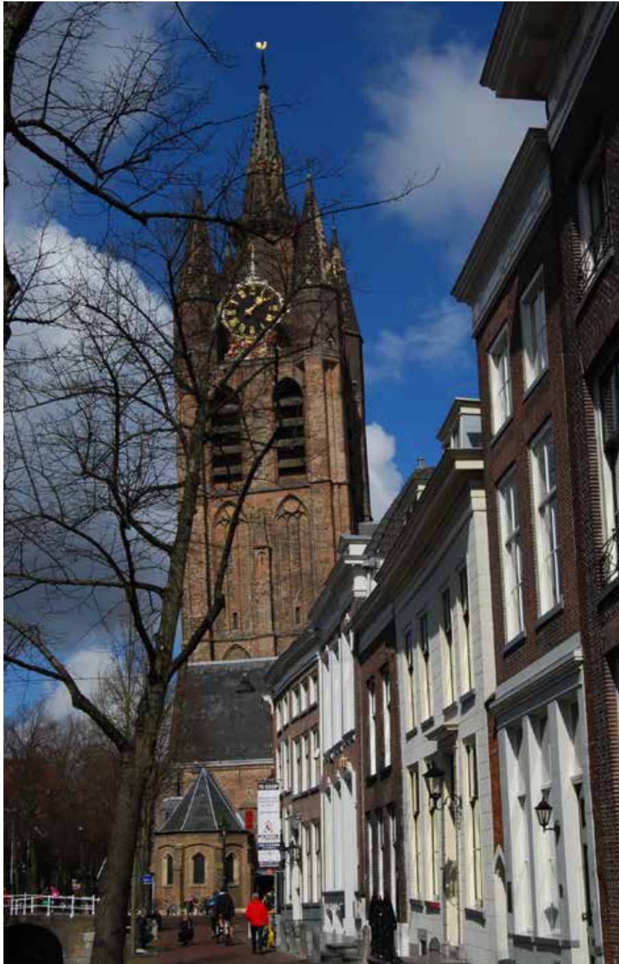
Figure 2.1 Tower of the Oude Kerk, Delft: tilt, example of a situation that already arose during the time of construction
