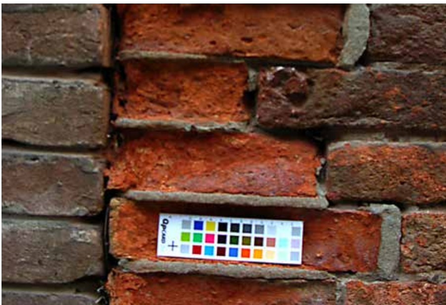
Figure 3.3.5 Incompatible re-pointing, resulting in accelerated damage to the brick
