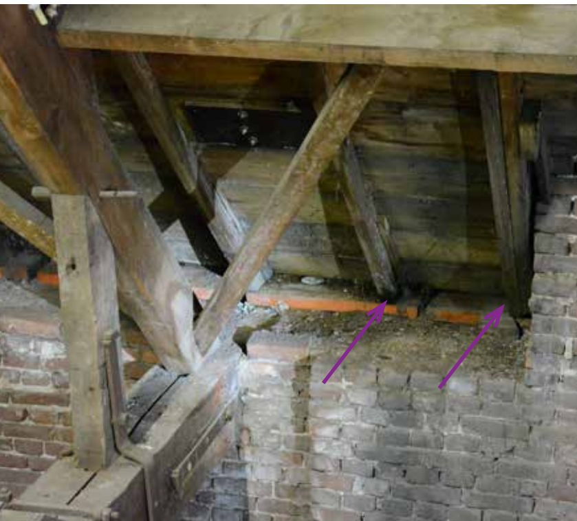
Figure 5.3a/b The consequential damage: the timber construction (see arrows) has become wet. Fortunately, the problem was approached immediately: tiles were replaced Figure 5.4 a/b/c Problem as encountered and improved situation at the connection be-
