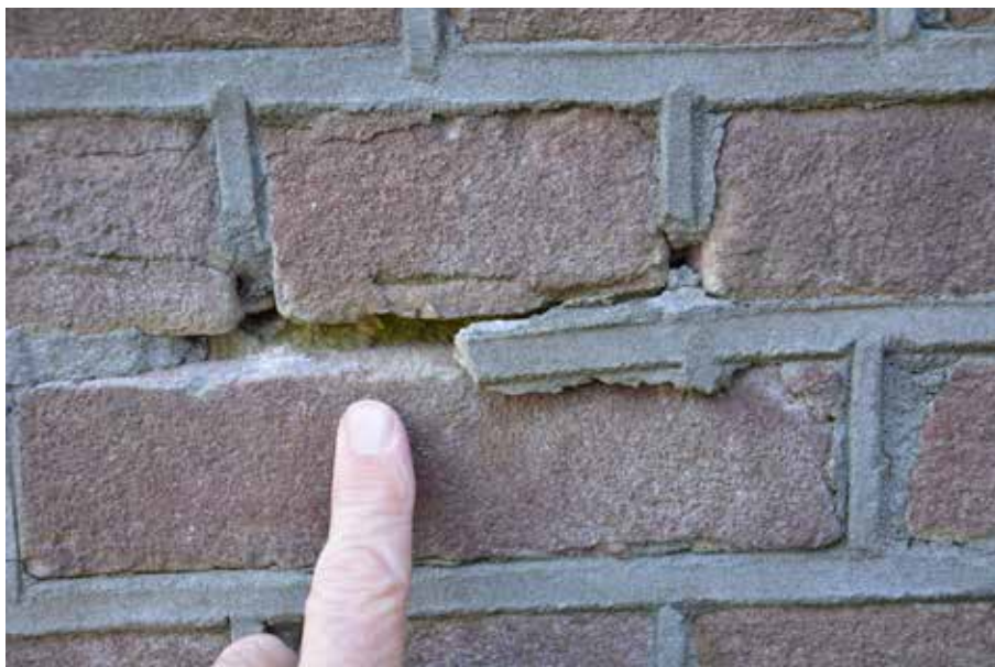
Figure 5.1 Pushed out pointing. Annoying, but it is a problem that can be tackled in the medium-long term
