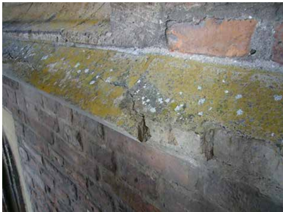
Figure 3.1.3 Loose part of a tuff stone cornice, in case the façade faces a public path there is acute danger for passers-by
