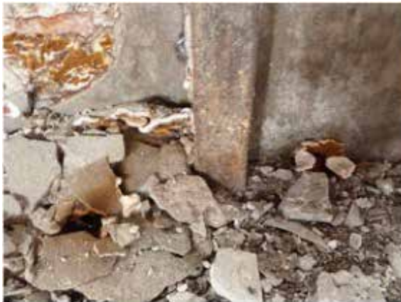
Figure 3.2.4 Dry rot fungus, spread between the plasterwork and the underlying masonry
