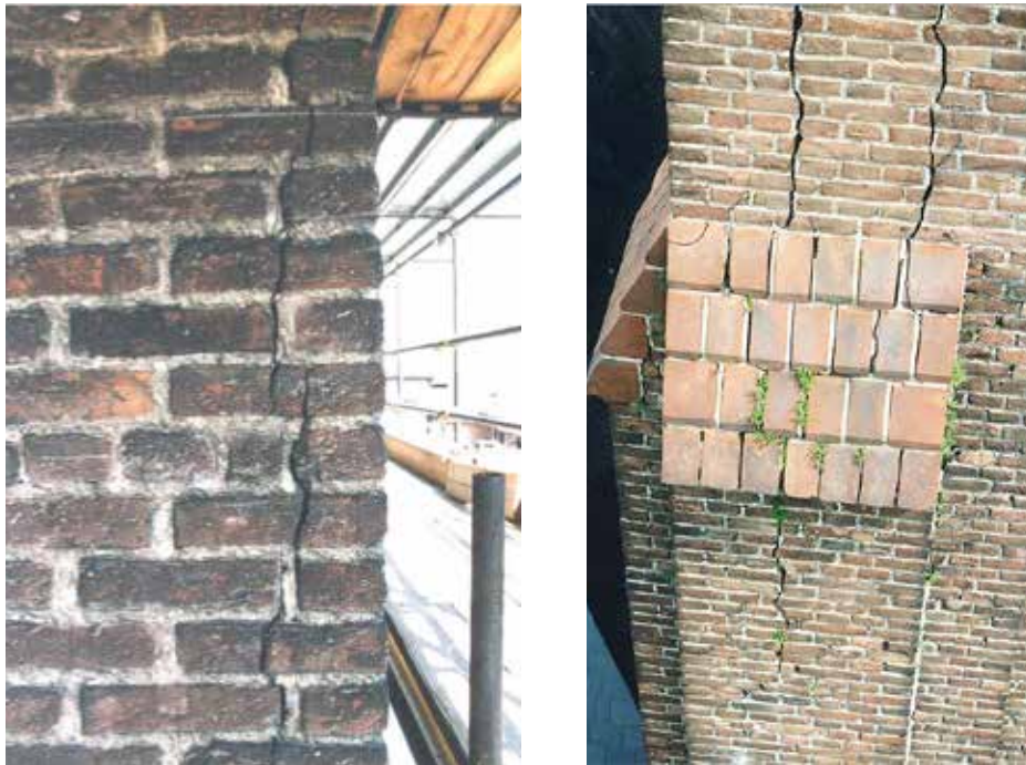
Figure 3.1.4 Comparable crack patterns. In the left case (detail of a tower in Italy) it was a structural problem that led to the tower collapsing. In the right case, laboratory investigations showed that the cracks resulted from a swelling reaction in the bedding mortar, used for the masonry behind the visible brick layers: a nasty problem, how-ever without the risk of collapse
