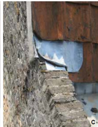
Figure 5.4 a/b/c Problem as encountered and improved situation at the connection between roof and façade (a. As encountered; b. Improved; c. Condition two years later)
