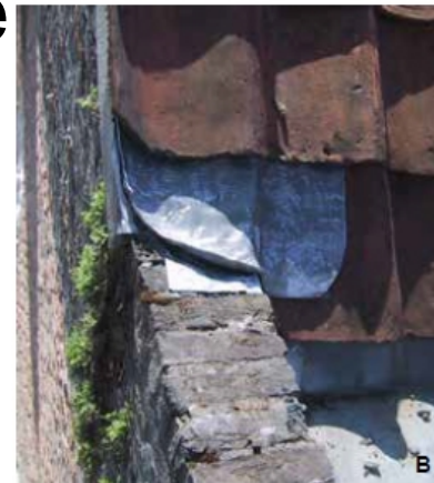
Figure 5.4 a/b/c Problem as encountered and improved situation at the connection between roof and façade (a. As encountered; b. Improved; c. Condition two years later)
