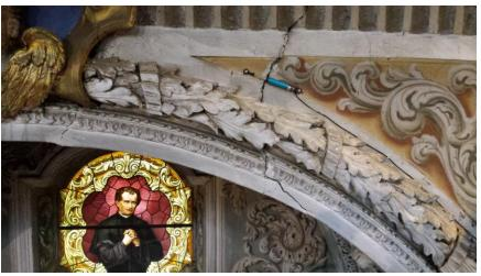
S. Maria church in Lovero displays a wide crack pattern: it was installed a structural monitoring system of the
