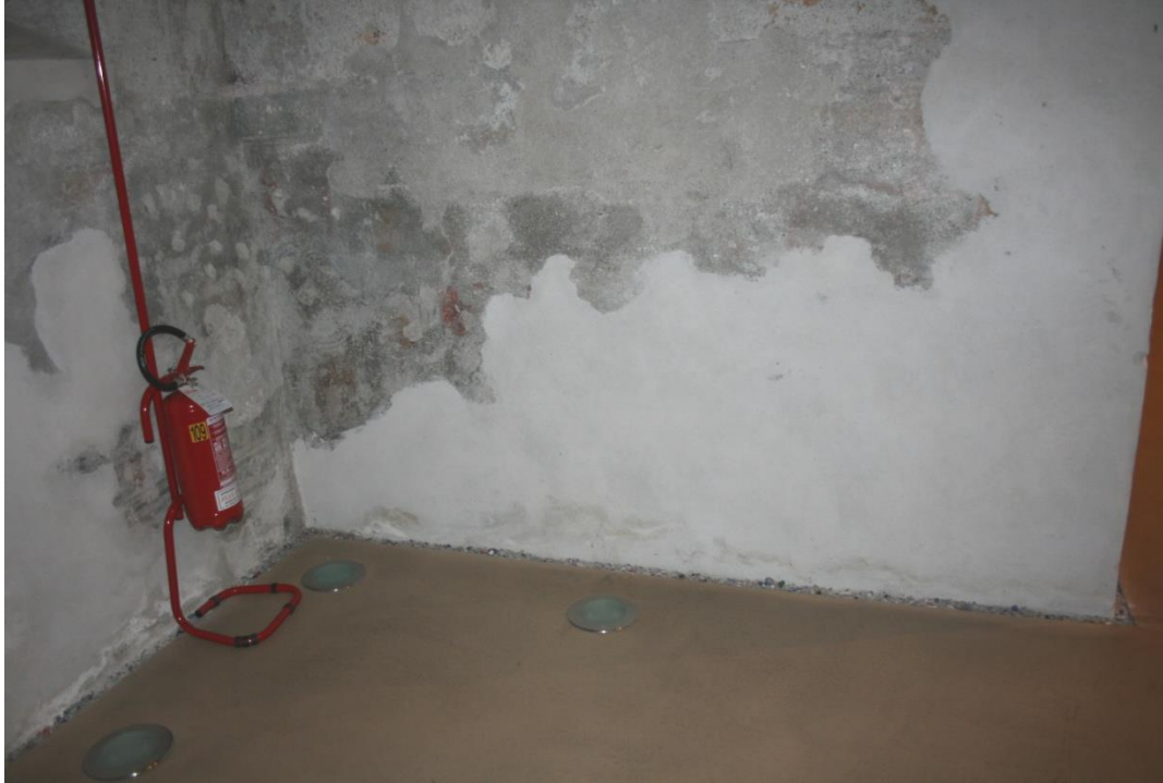
Auditorium: humidity and efflorescence on the low plaster, beside the frescos (first left chapel)
