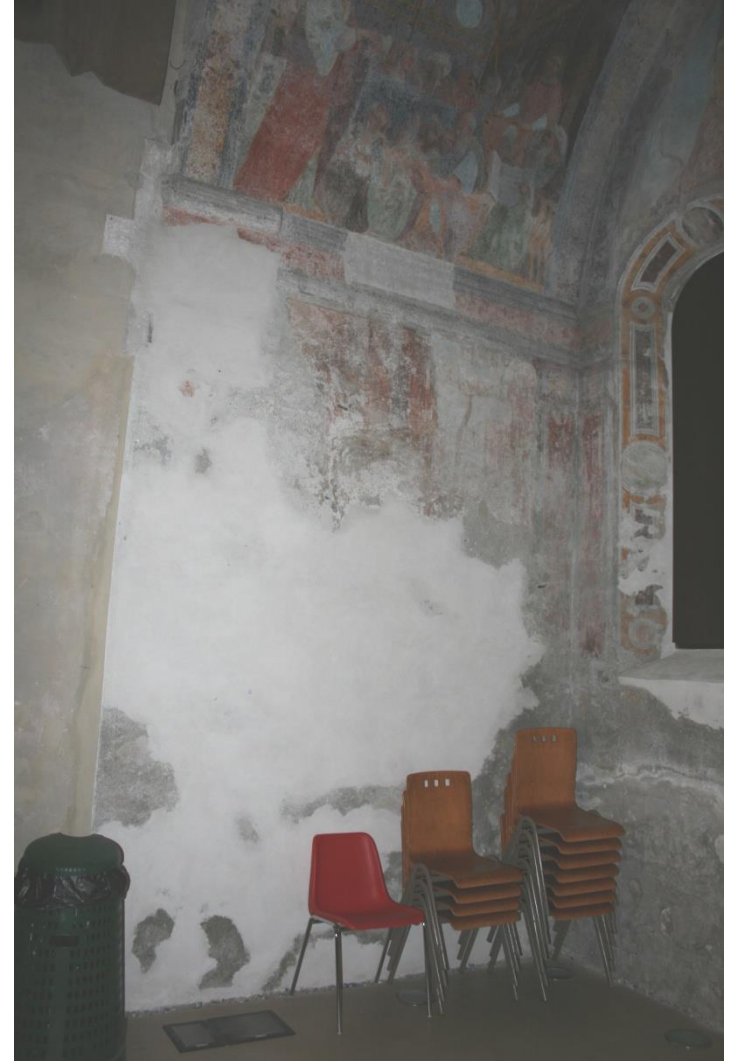
Auditorium: humidity and efflorescence on the low plaster, beside the frescos (first left chapel)
